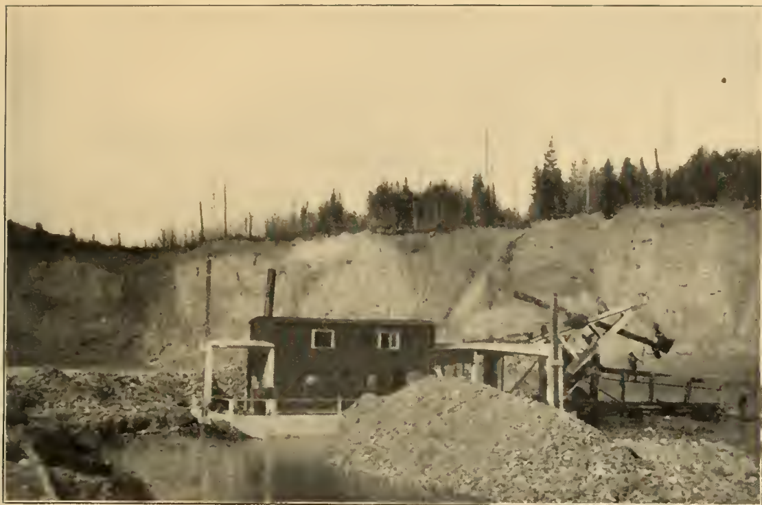
NEWALL DREDGE—CUTTING THROUGH BAR—FRASER RIVER.
